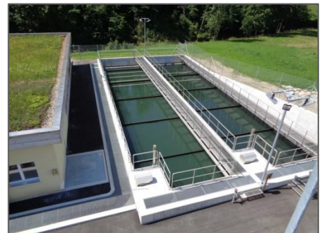
Sedimentationsbecken PAK-Stufe (links Filter)
